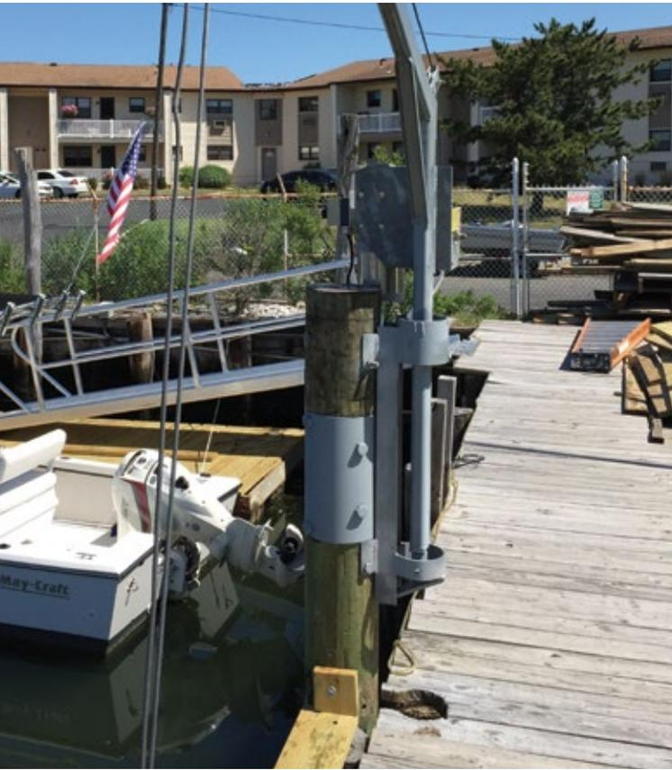
LoClear Piling Systems performed engineering testing on similar splices and achieved lateral loading of five tons before failure. A virgin 10-inch butt pile also failed at five tons when subjected to a similar test.
